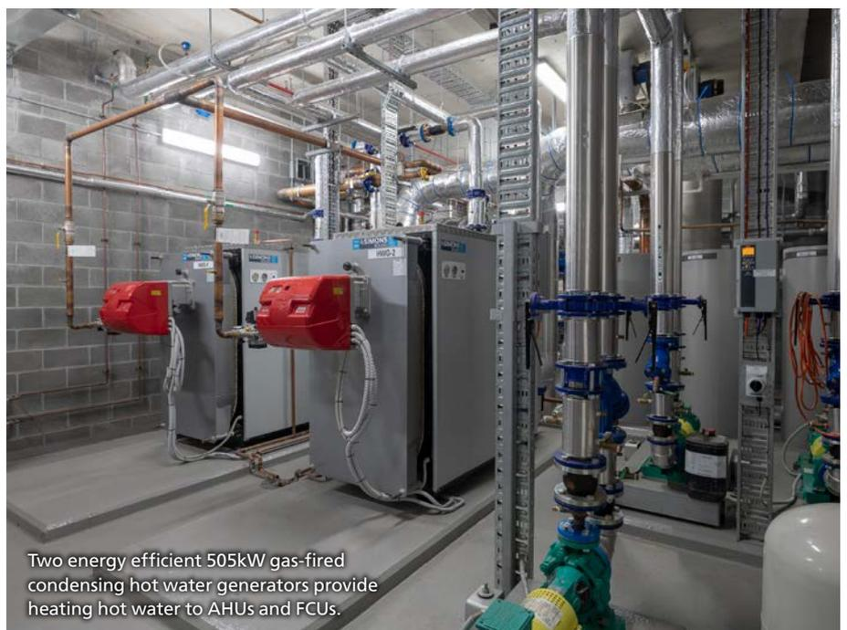
Two energy efficient 505kW gas-fired condensing hot water generators provide heating hot water to AHUs and FCUs.
