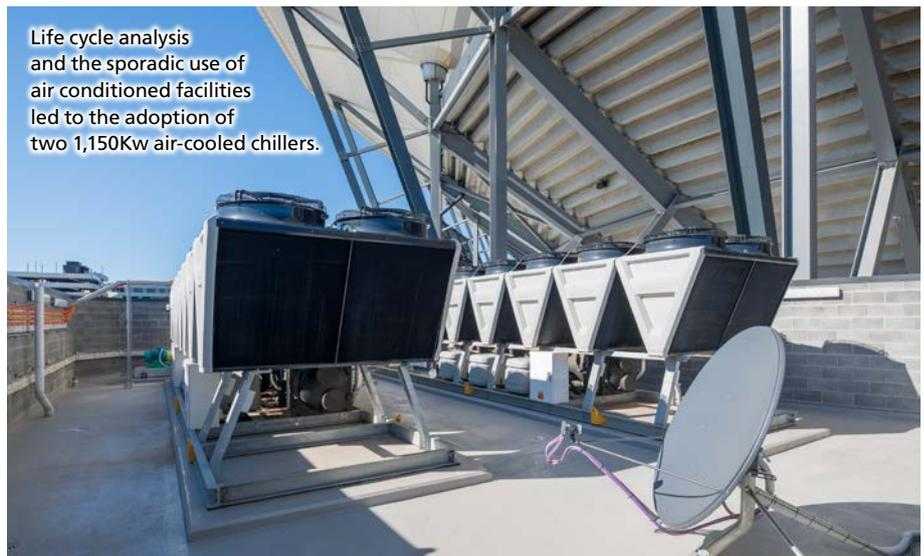
Life cycle analysis and the sporadic use of air conditioned facilities led to the adoption of two 1,150Kw air-cooled chillers.
