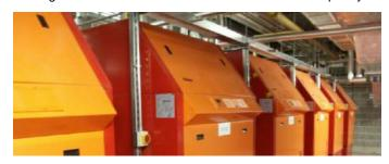
**Maintenance:** The 'dry' combustion side of the heat exchanger requires oxidised deposits to be brushed off and then cleaned away. If this is not regularly carried out, deposits will block the neutralising trap and cause condensate build up in the heater. This will ultimately result in ignition failure (nuisance tripping) and corrosion of the unit.
