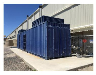
40 foot shipping container adapted for use as a mobile boiler plant room.
